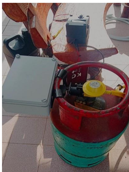
Figure 5. Installation of The Project
