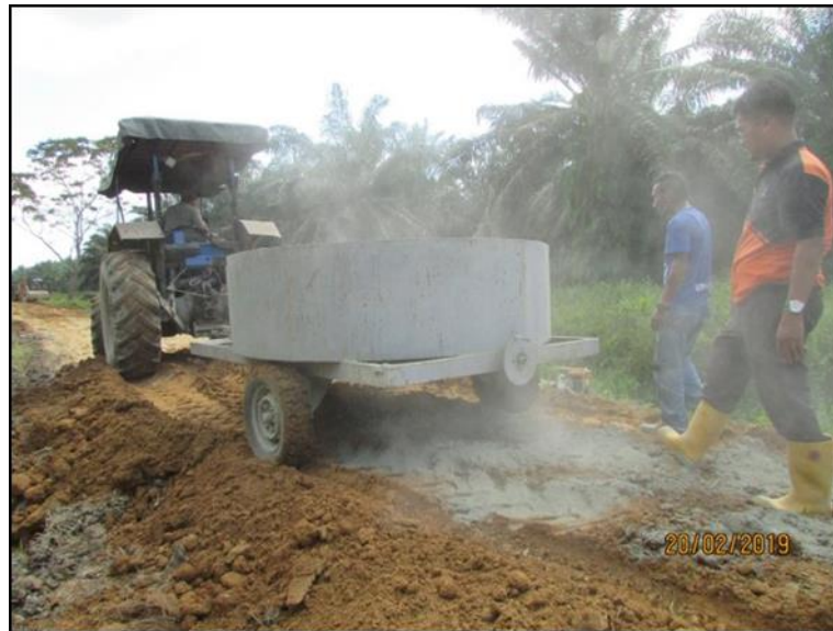
Figure 3. A custom-made pan mixer.
