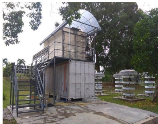
Figure 1. Rooftop garden structure
